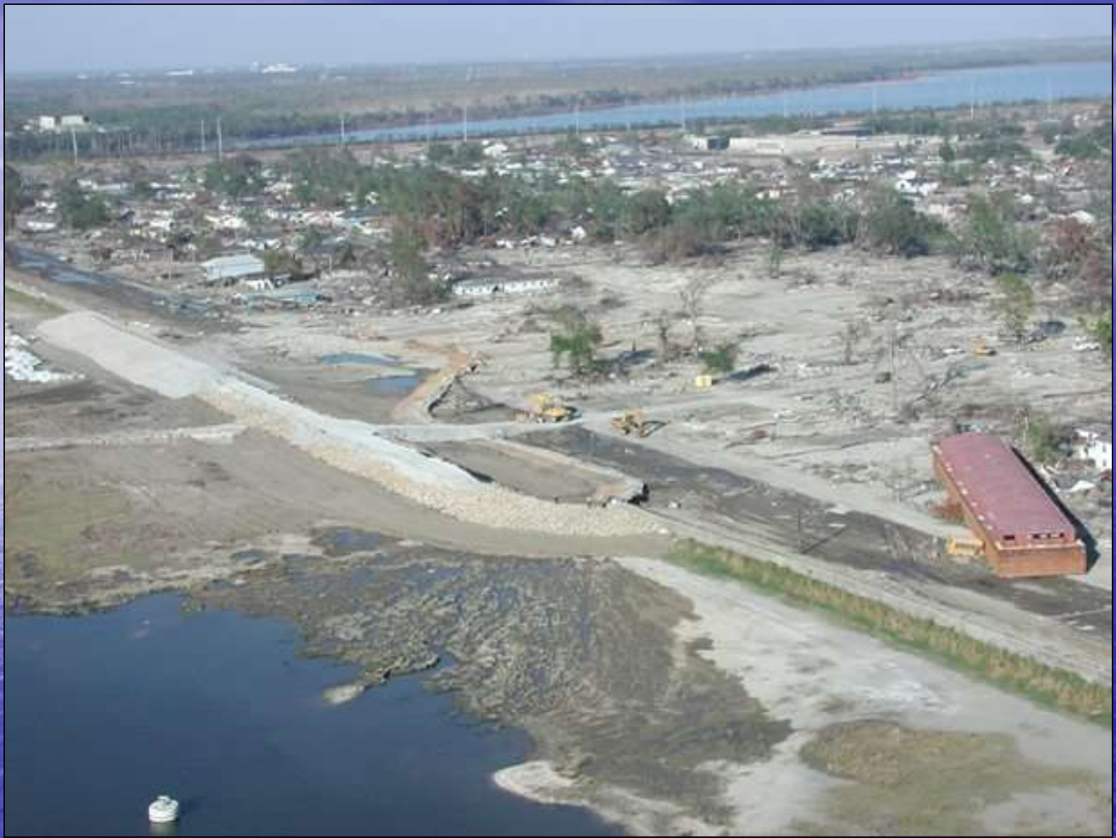
Seepage crevasse exposed at the east levee of the IHNC breach after Hurricanes Katrina and Rita
